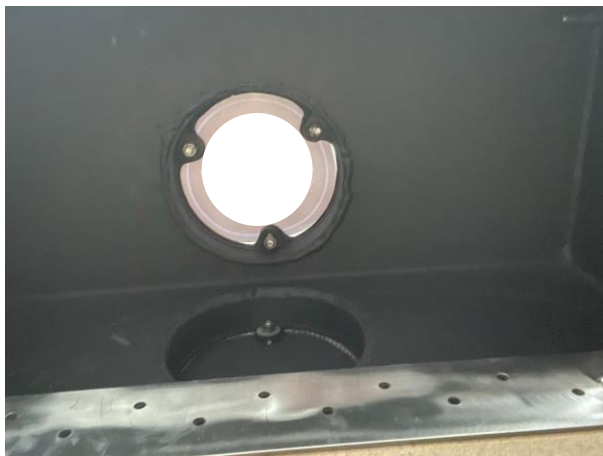
6. Remove baffle through door opening at 45° to reveal access to flue for sweeping.
