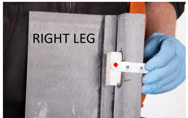
● FIX TO BLOCK ON OUTER RETURN – POSITION INDICATED ON PICTURE TO LEFT (SCREW AND RAW PLUG INCLUDED)
